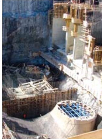
Construction on the Wuskawatim generating station dam.
